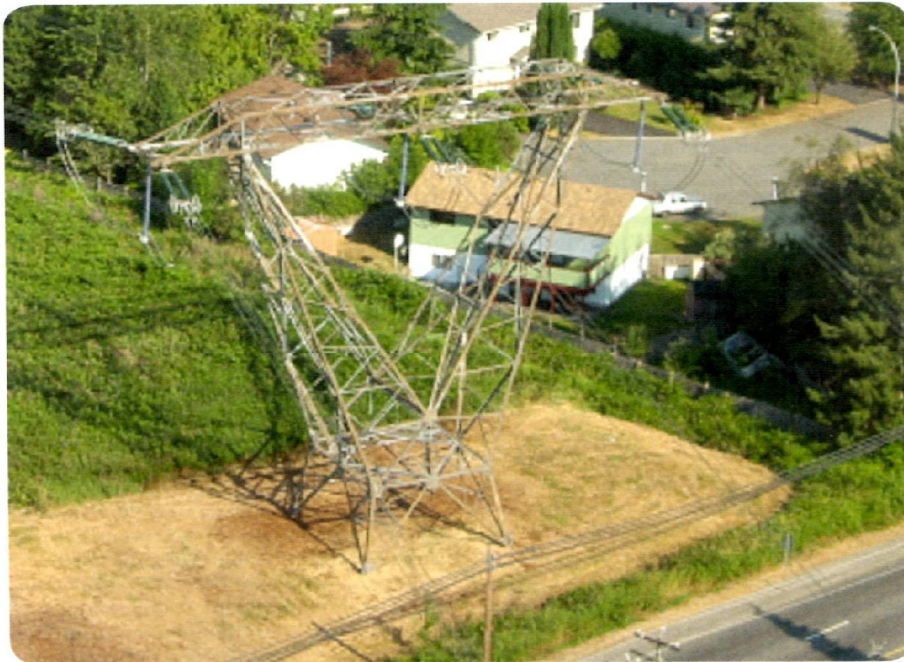
FIGURE 2 Utility transmission and distribution towers located in environments where land use (e.g., proximity to industry, roads, and deicing salts) is indicative of potential corrosion issues.
